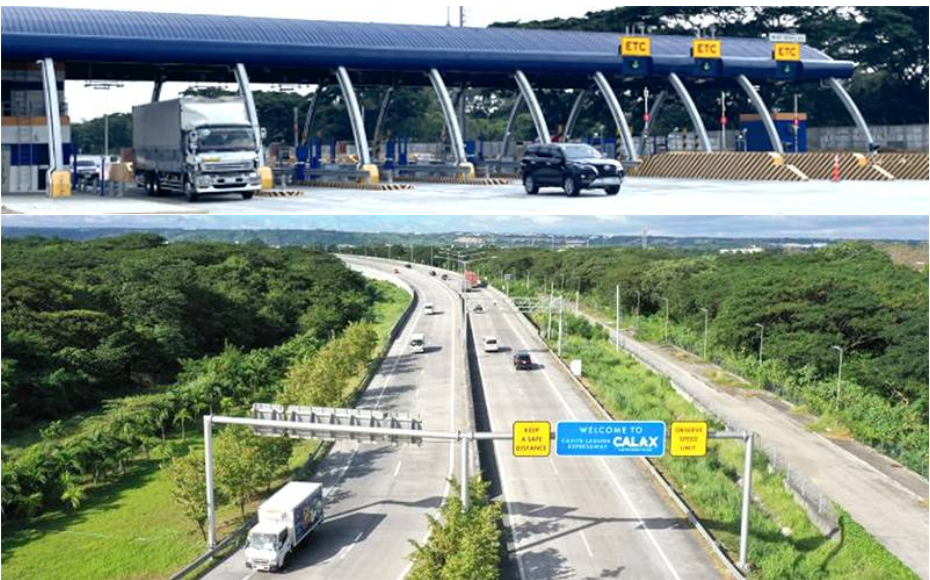
The economic landscape of Cavite is poised for greater growth following the opening of the Cavite-Laguna Expressway (CALAX) Subsection 3, extending the expressway to Governor's Drive Interchange in General Trias City.
